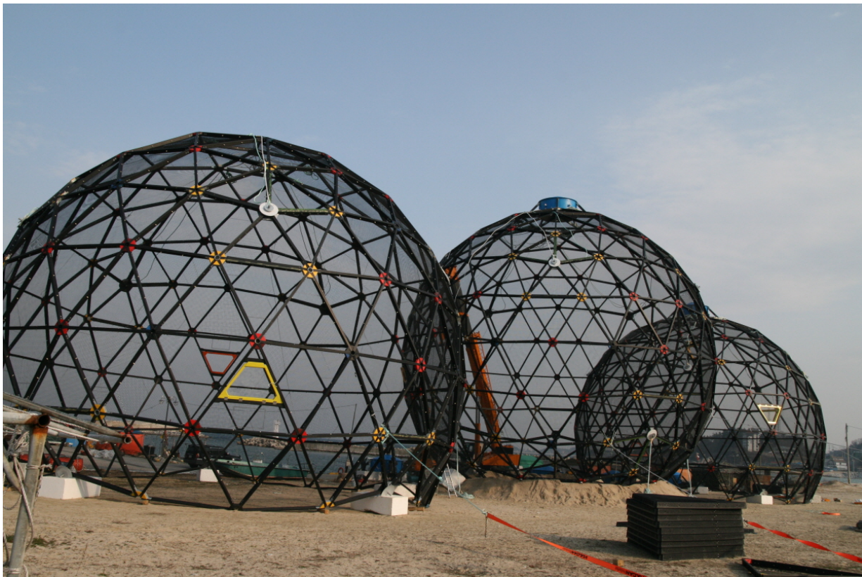
Three A3600 Aquapods during assembly in Yangyang, South Korea.
