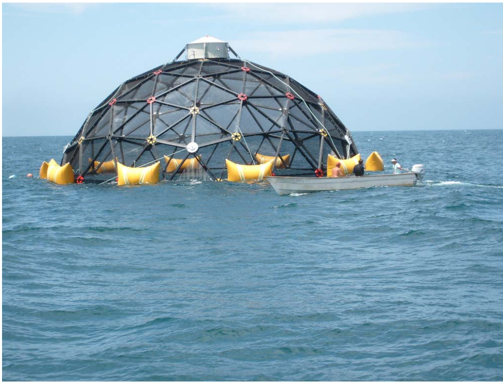
An A3600 Aquapod during installation in Guaymas, Mexico.
